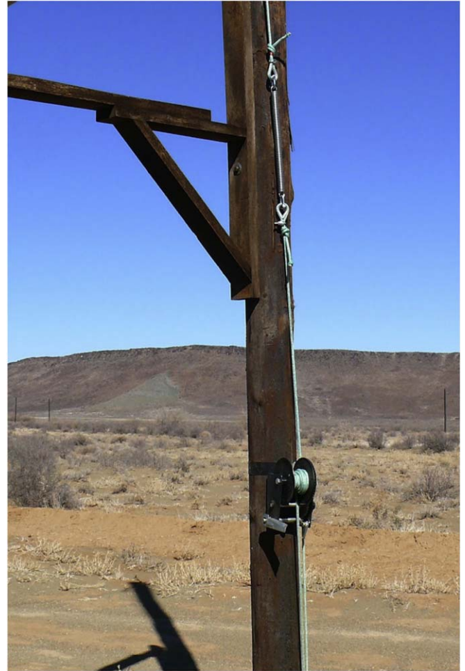
Figure 10. The feeds are raised and lowered with a hand winch. Each pole serves 3 surrounding antennas, therefore each pole also supports 3 winches, except for edge cases such as the one in this figure. Also visible is the extension spring which allows safe adjustment of tension force. Originally these were located at the feed attachment point, but were observed to introduce notable distortions in antenna response.
