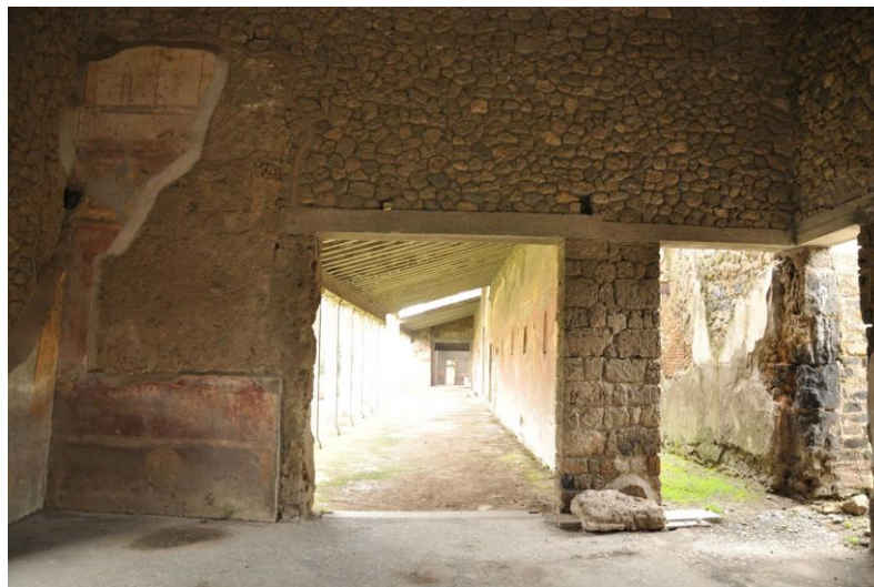
Figure 7.13: Portion of the wall with frieze
