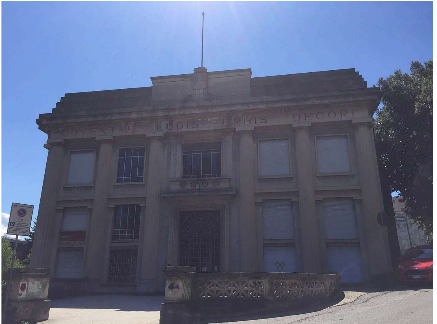
Eastern façade of the Palestra XXV Aprile, facing Via Guido Morselli
