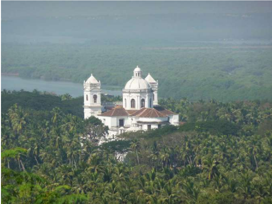
Figure 1 – Church of Our Lady of Divine Providence, Goa, India (credits: Sidh Losa Mendiratta, 2020).
