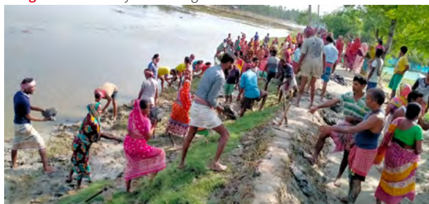
Image 2. Community Rebuilding of an Embankment After a Breach
