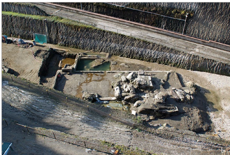
Fig. 2. a) Plan of the recent excavations; b) Aerial view of the collapsed monumental hall of the Villa dei Papiri (courtesy of Maria Paola Guidobaldi).
