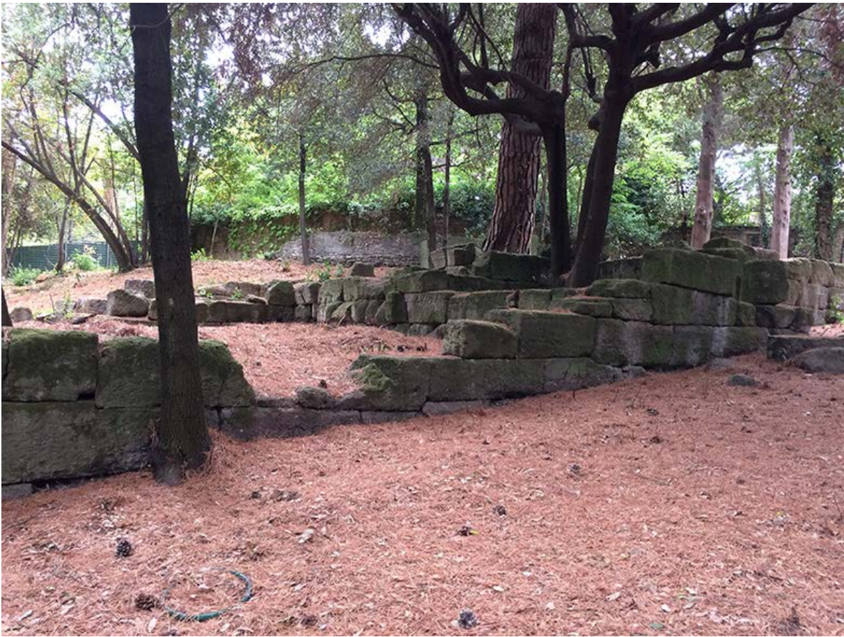
Fig. 16. Building in opus quadratum , seen from the SW (2017).
