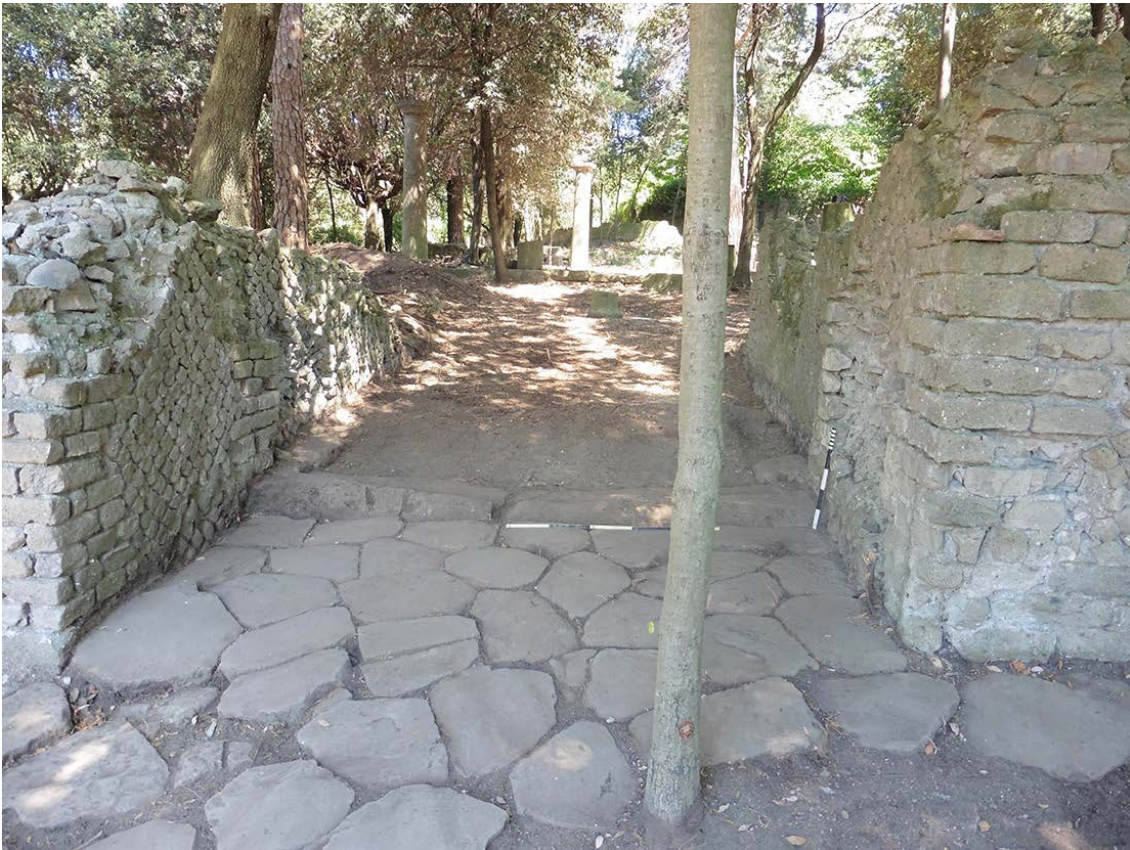
Fig. 7. Entrance S with threshold in peperino seen from the south (2017).
